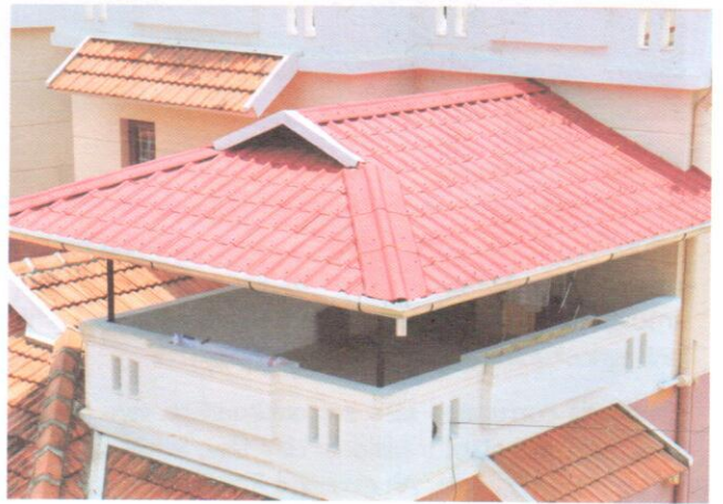
Terrace covering (Tiles)
